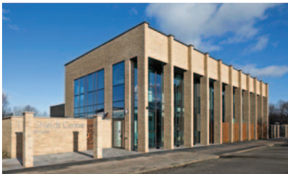
The Shields Centre, Glasgow.
