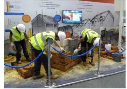
Apprentices from Grangewood Brickwork Services building demonstration corner details in brick and blockwork at Ecobuild 2016.
