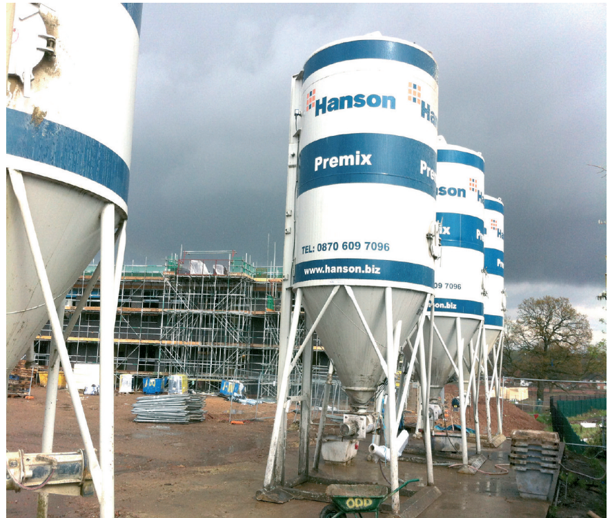
Five silos on site ensure readily available mortar supplies
