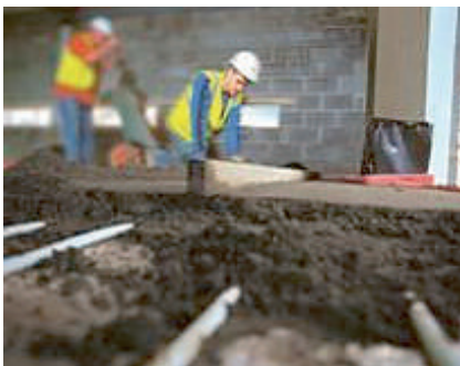
Laying a cementitious floor screed
