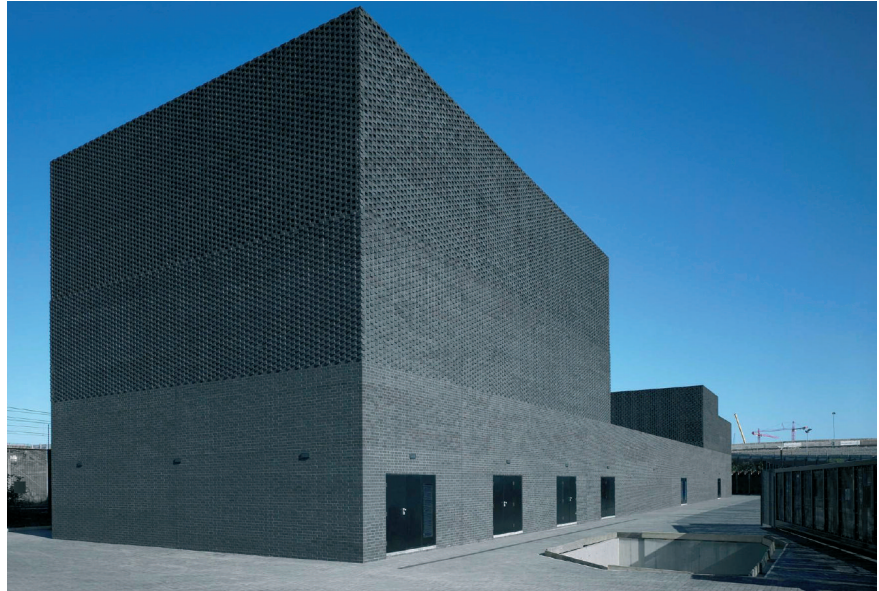
The substation at the London 2012 Olympic Park
