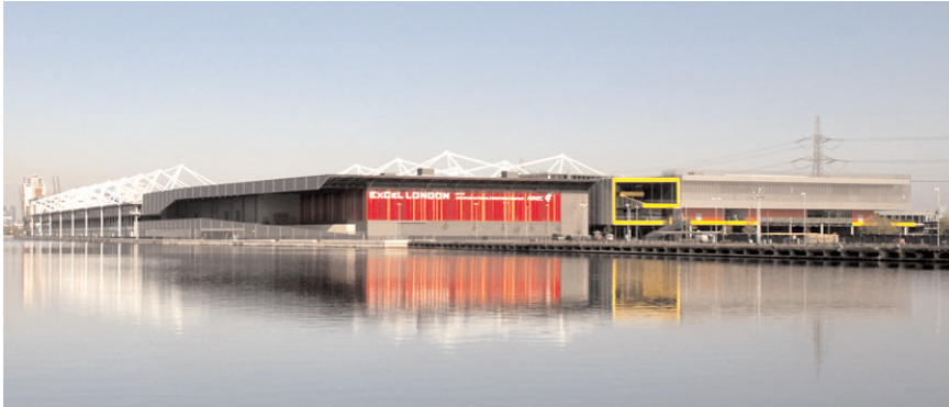
General view of the extension to the ExCel Centre
