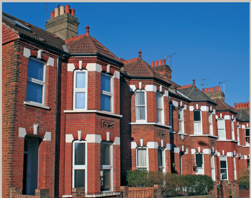
Twenty-five per cent of UK housing stock is of solid nine-inch brick construction.
