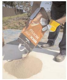
Ready mixed dry mortar is produced in 25kg bags and where these are stored on site it is essential that they are covered and stored in a dry environment.
