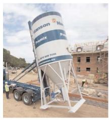
Silos are not usually delivered full because the gross weight would be in excess of statutory legislation. They are subsequently filled on site by blowing in refill material from a tanker.
